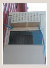
Optional enclosure roof and temperature-controlled ventilation system with emergency back-up power supply.
