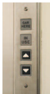
Above control station only available with bi-parting and slide-up doors.
