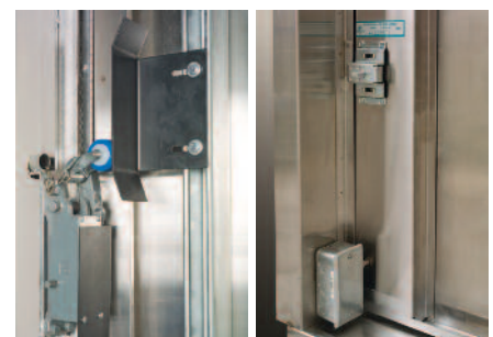
Car cam and roller position shut-off switch meets all industry codes as a dumbwaiter door safety interlock.
