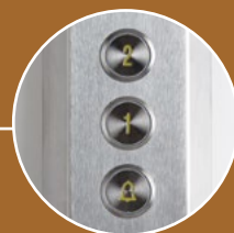
Cab Operating Panel, with Hall Station at each landing's door
